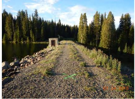
Figure 1. Dam crest and B-102A prior to drilling activities, looking south. Green "X" in photo indicates boring location.
