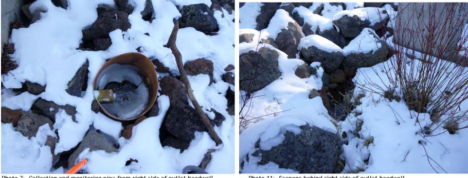
Photo 7: Collection and monitoring pipe from right side of outlet headwall.
