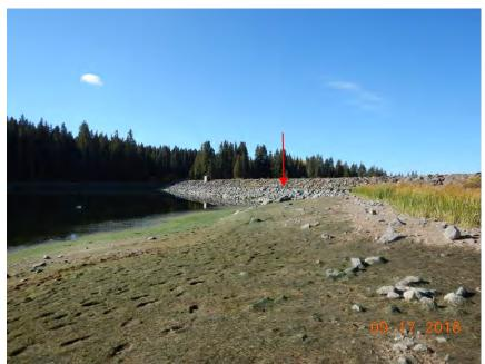
Figure 5. Carson lake water level prior to drilling activities, looking southwest. Water level is about 10 feet below normal maximum. Normal maximum marked with red arrow.
