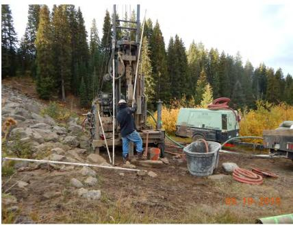
Figure 2. B-105A during monitoring well installation, looking south.
