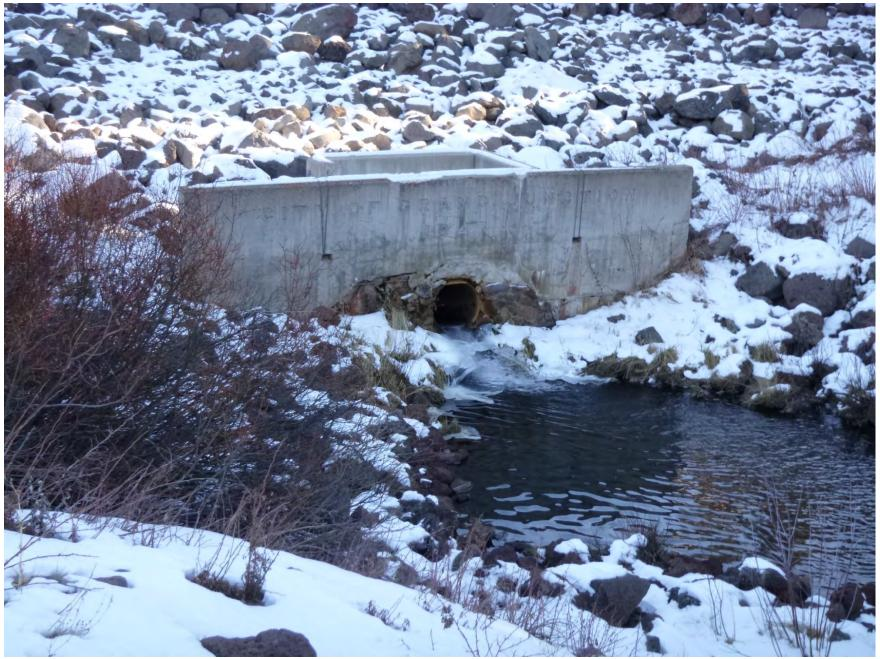
Photo 5: Downstream outlet pipe headwall.
