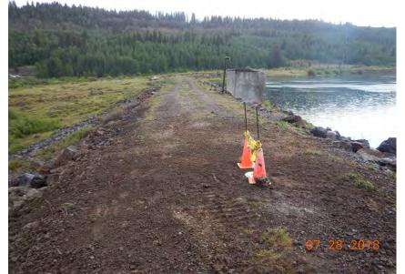
Figure 3. B-101 at end of day, looking north. Cones and caution tape placed either side of monitoring well surface mount casing.
