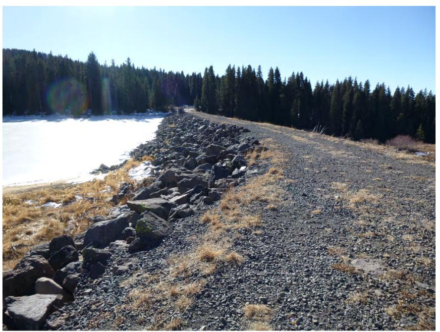
Photo 2: Upstream slope; Outlet hydraulics control building at center of dam on upstream edge of dam crest.
