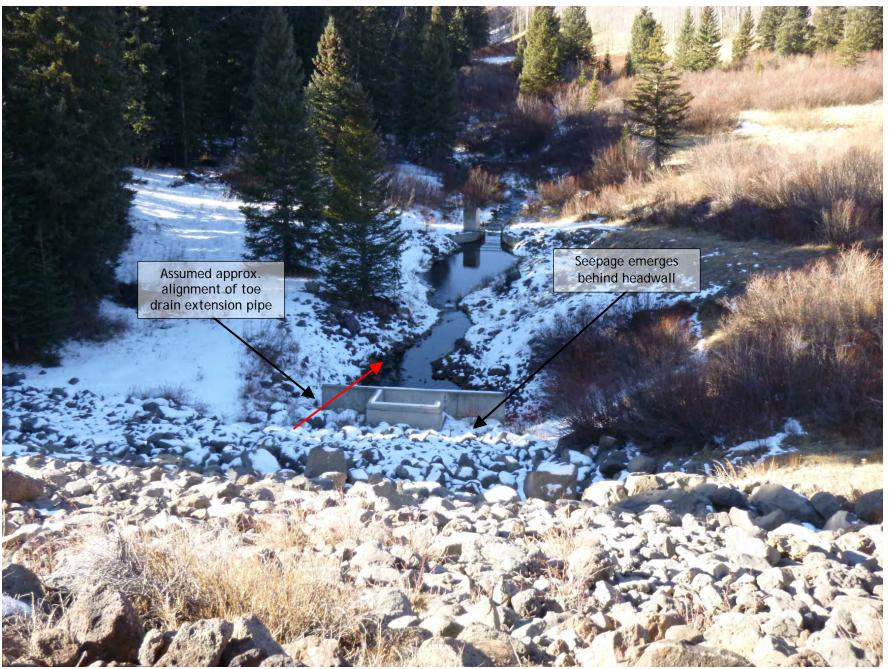
Photo 4: Downstream outlet headwall.
