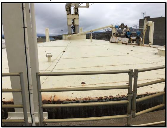
Picture 33 Anaerobic Digester Tank Roof (floating lid)
