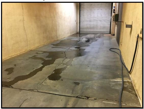
Picture 25, Aerobic Digester Concrete and Wall Cracks (Truck Sludge Loading)
