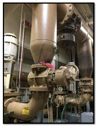
Picture 16, Aerobic Basin Basement Pump Pipe Erosion at Reducer Flange
