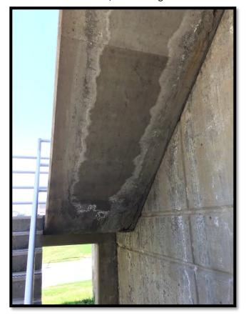
Picture 24, Aerobic Digester Stairway, Rebar erosion in concrete
