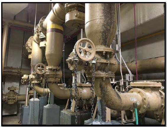
Picture 17, Aerobic Basin Basement Pump Pipe with spray from reducer leak
