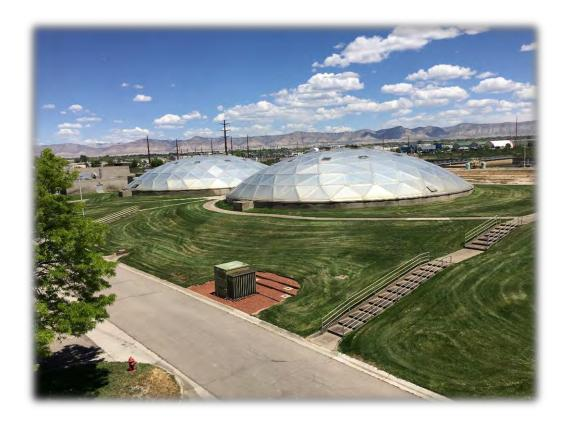
Each primary clarifier is115 feet in diameter. Settleable wastewater solids are removed by these units by gravity settling. A scraper mechanism collects and moves the solids to the center of each clarifier where they are drawn off and pumped to anaerobic digesters for further processing.
