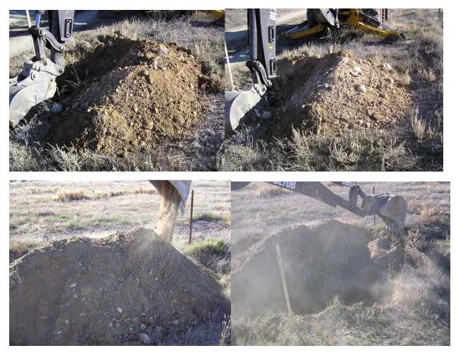
The top 1 foot was generally consistent with that of a sandy clay (CL) material. 1 - 4 feet the material was a pit run, cobble material (SM). 4 - 7 feet the material turned to a decomposed shale material.
