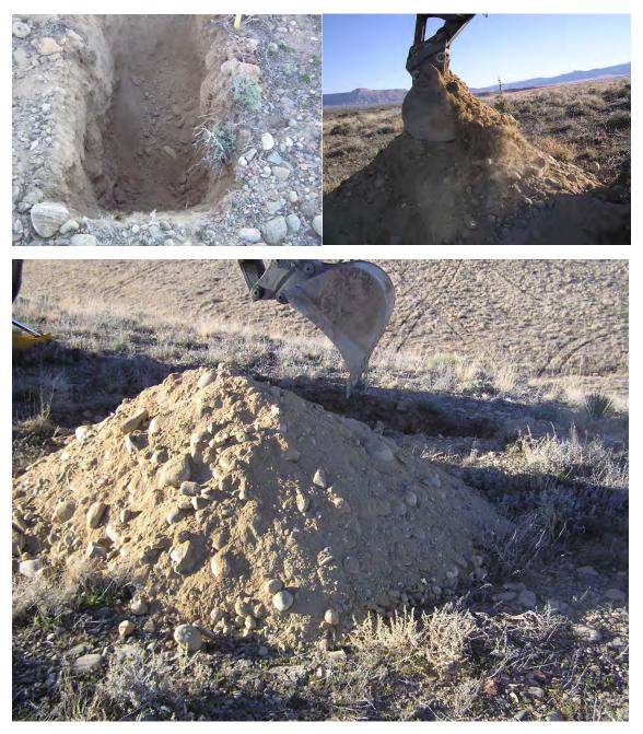
The full depth of the test hole to 5 feet consisted of pit run cobble material poorly graded with a sandsilt mixtures (SM). Test hole #4 approximate station 63+38, Center location of the proposed water tank
