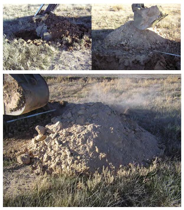
The top 1  $\frac{1}{2}$  foot was generally consistent with that of a sandy clay (CL) material. 1  $\frac{1}{2}$  - 4 feet the material was a very fine sand /rock flour material (ML).
