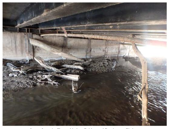
Large Logs in Channel below Bridge and Resting on Girders
