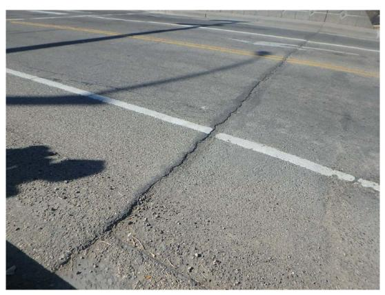
Transverse Crack in Asphalt Typical along Top of Abutments
