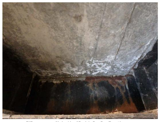
Efflorescence on Underside of Deck in Bay B at East Abutment
