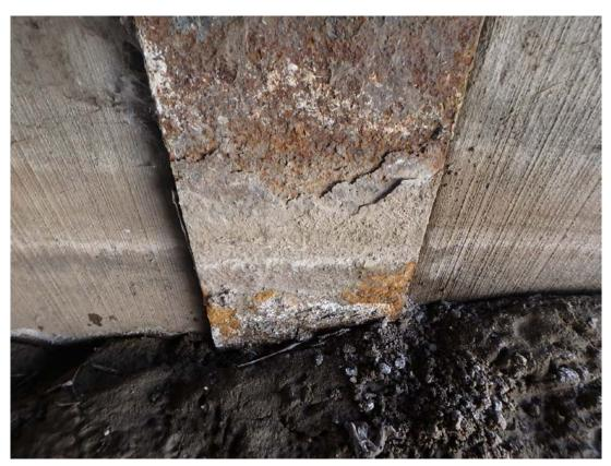
Typical Flaking Rust on Exposed Flange of Abutment Pile
